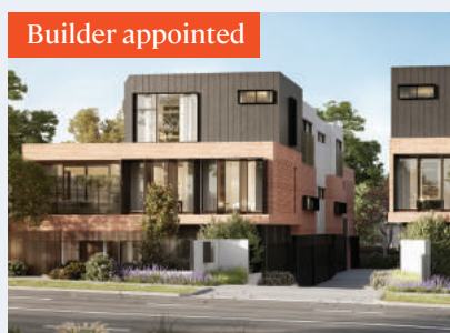
Builder appointed BURTON PLACE Ashburton
