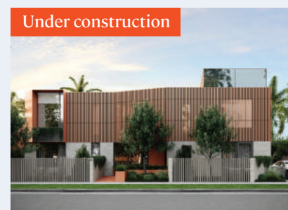
Under construction CASA ELWOOD Elwood
